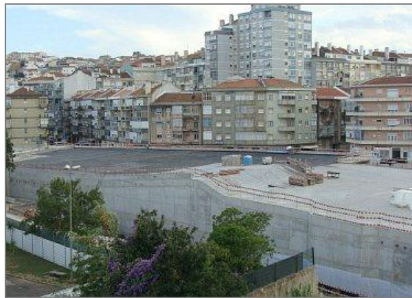
Figure 2: The CRIL during construction (Source: www.cril-segura.com )
