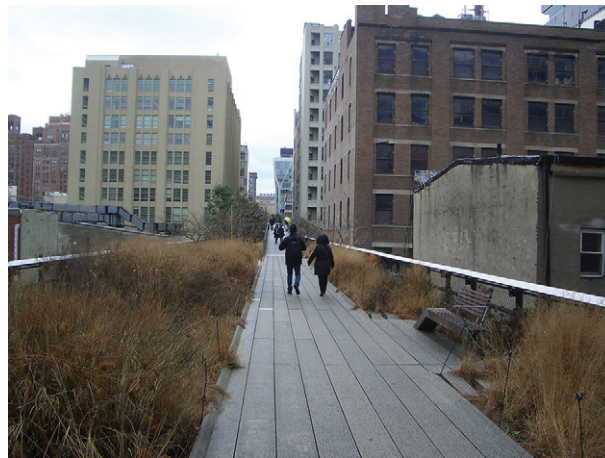
Figure 5 Example of reconversion of elevated transport infrastructure (New York, United States).
